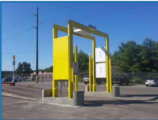
Up to four detector systems (lanes) can be networked together via Ethernet or wireless to the central PC where vehicles entering from either direction can be monitored in real time. Each detector system additionally includes a remote control/annunciator panel to support operator awareness, alarm acknowledgement, and if necessary, backup operation in the event the central PC is unavailable.
